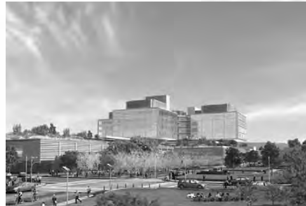
View of the New Stanford Hospital from Welch Road
